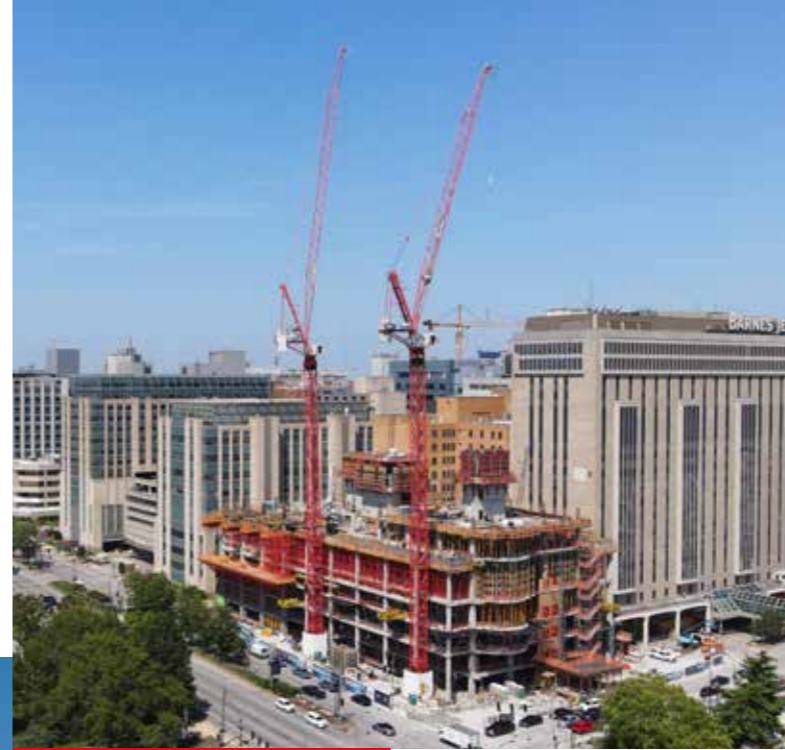
BJC Campus Renewal, St. Louis, MO, USA
